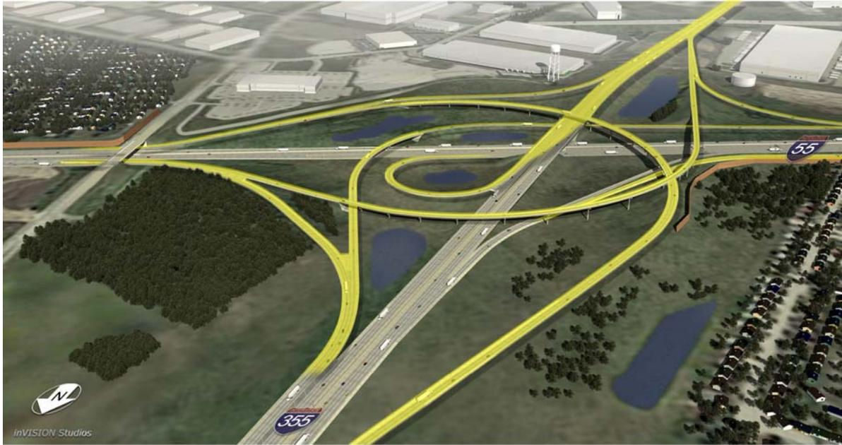
Work began in spring 2006 at the site of the new I-80 interchange at Cedar Road, which features four ramp movements at the southern terminus of the roadway, including two flyover ramp bridges. The flyover ramp movements are for southbound I-355 traffic heading to I-80 eastbound and for eastbound I-80 traffic heading northbound on I-355.
